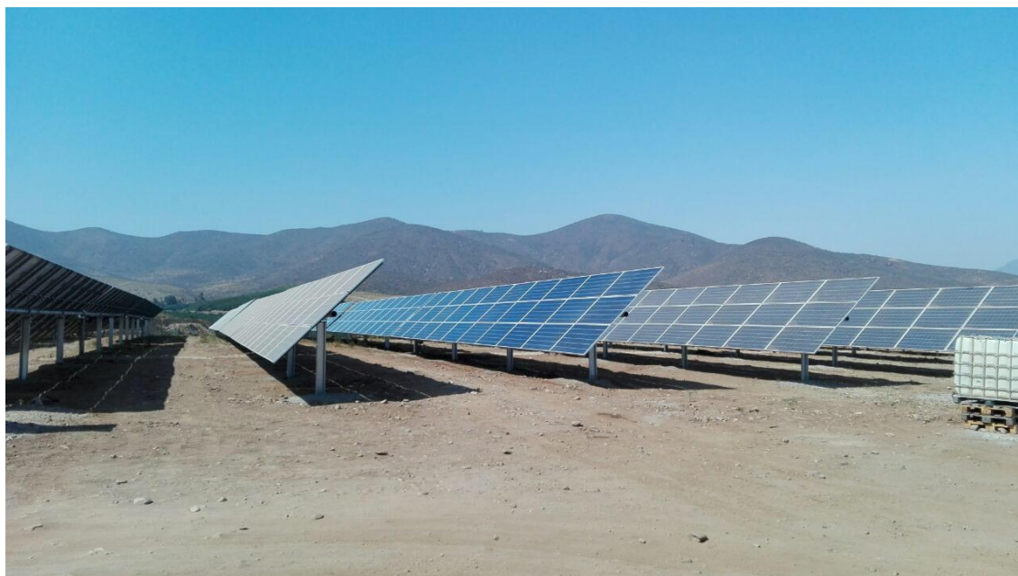
Fig. 3 The PV power plant in Chile with movable stands of PV panels with solar trackers and with horizontal axes
