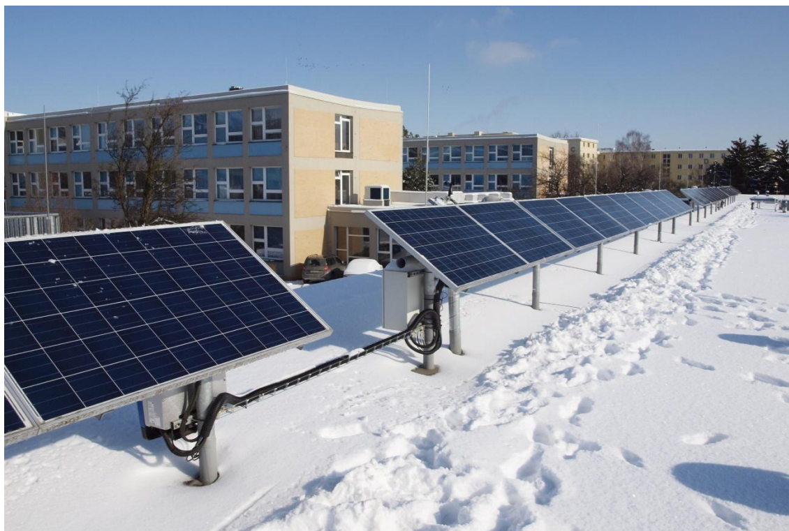
Fig. 4 The PV power plant in Prague at CULS with fixed stands of PV panels with inclination 35^\circ to the south
