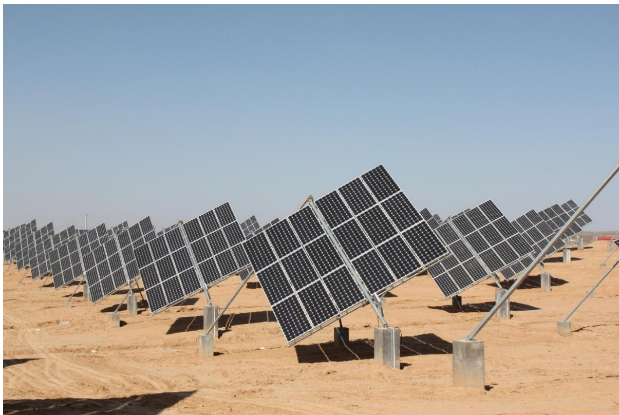
Fig. 1 The PV power plant with tracking stands TRAXLE of PV panels
